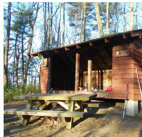
Helveys Mill Shelter
